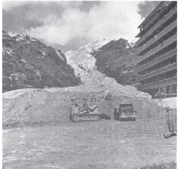
Figure 17. Debris from Type 1 slip, decomposed granite fill
