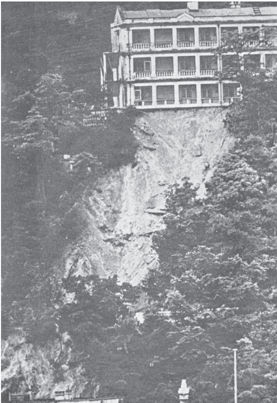
Figure 16. Type 1 slip, platform
