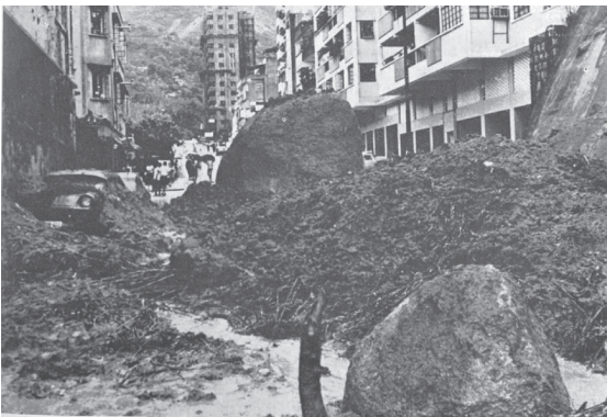
Figure 19. Debris from Type 2 slip, decomposed granite
