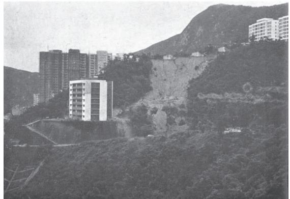
Figure 18. Scar from Type 1 slip, decomposed granite fill
